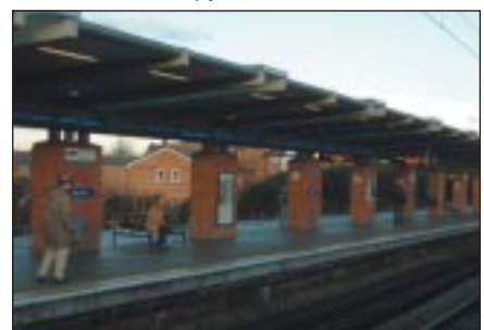
West Ham – in comparison, much better sign frequency on the Underground platform
