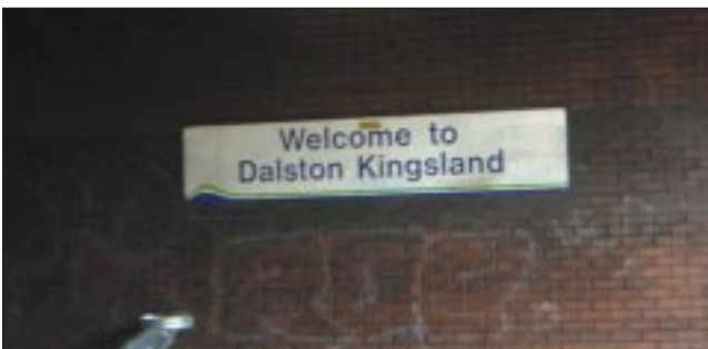
Sign size is 3000mm x 600mm 1780mm from ground to bottom of sign
