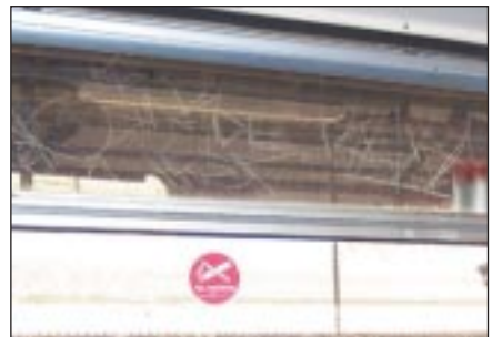
Clapham Junction – sign is difficult to read because of glare and shadow, and due to scratches on the window
