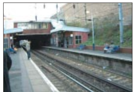
Dalston Kingsland (Silverlink) – three car platform. Three signs spread over 68 metres
