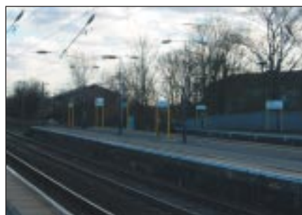
Mill Hill Broadway (Thameslink) – four platform with sign staggering (see section 4.1.3)
