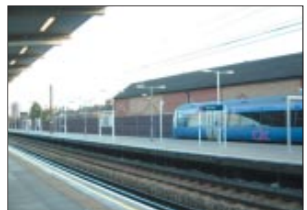
West Ham (c2c) – 12 car platform. 11 signs spread over 242 metres
