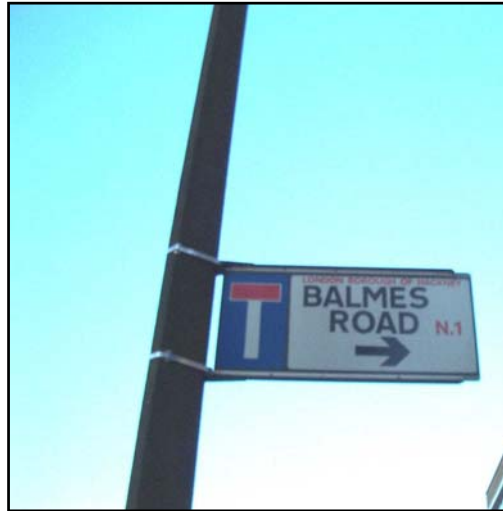
Double-sided nameplate attached to lamp columns also includes the no-through road sign in a location that is very visible all travellers, L B Hackney.
