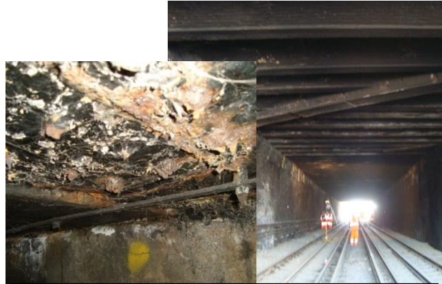
Highbury Corner - replace the road-over- rail bridge
