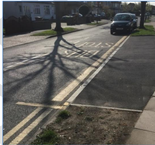
Right: Work to convert the Hail and Ride section on route B13 in Blackfen to fixed bus stops began in the first half of 2019. At the time of viewing, the clearway line, bus stop cage and correct kerb were all in place but the bus stop and flag were still to be added.
