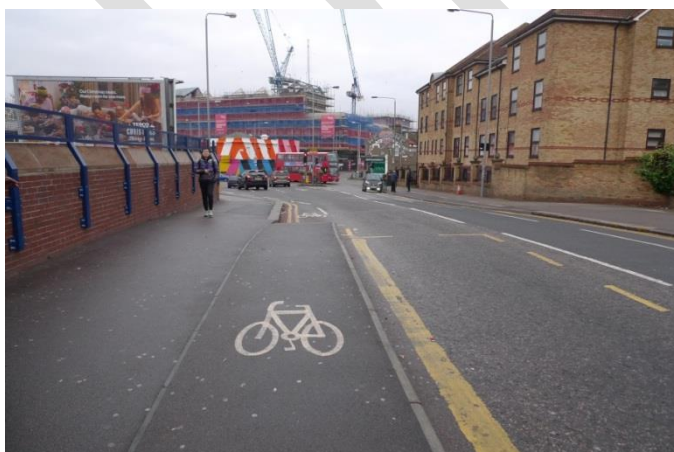
Figure 25. The approach to Forest Road on Blackhorse Road.
