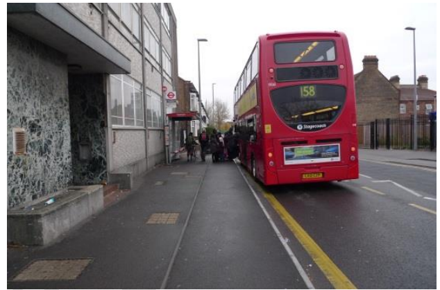
Figure 30 The cycle lane passes through the passenger boarding and alighting area
