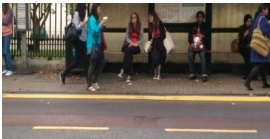
An inaccessible bus stop – the kerb height is too low for the bus ramp to properly reach the pavement, making it difficult for wheelchair users to get on or off the bus
