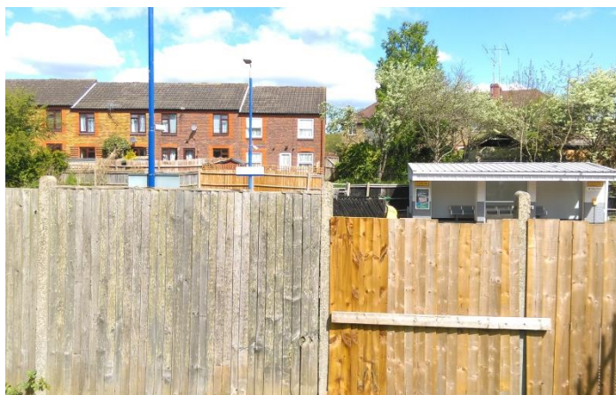
There is potential to provide step free access to Sudbury Hill Harrow station from Hartington Close
