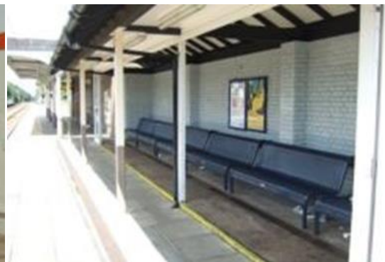
Step up to sheltered seating area on platform 1
