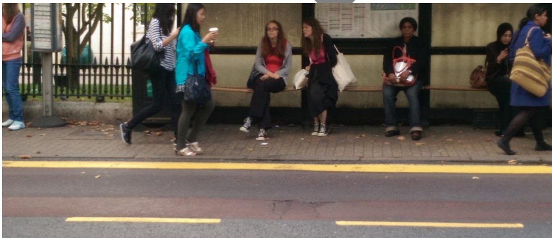
Figure 1: An inaccessible bus stop – the kerb height is too low for the bus ramp to deploy properly.
